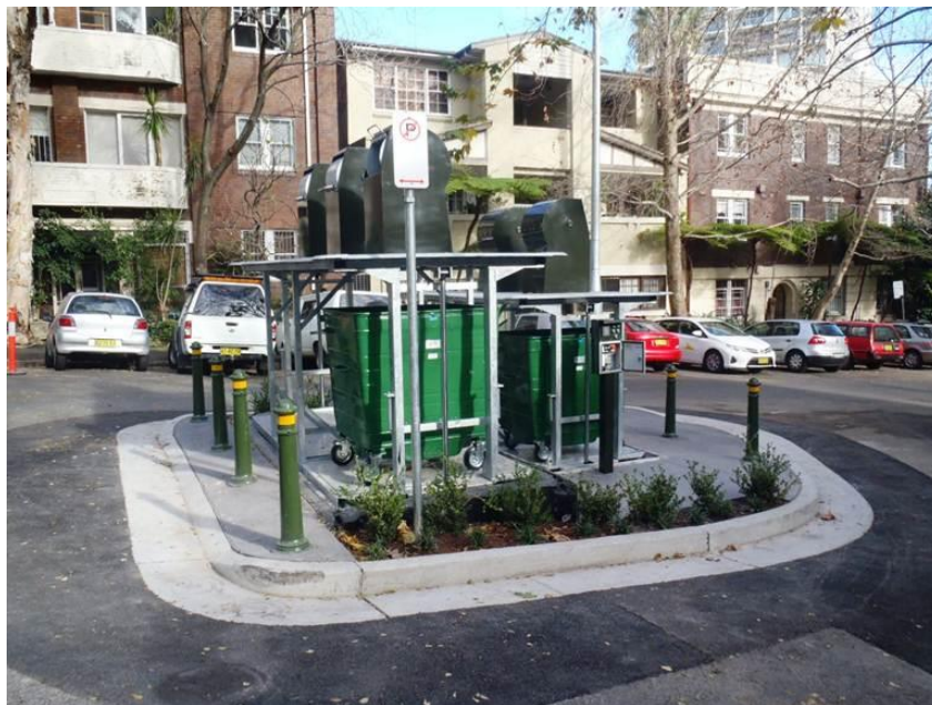
Figure 31 - Hydraulic-underground bins at Royston Street, Darlinghurst (Sydney)
