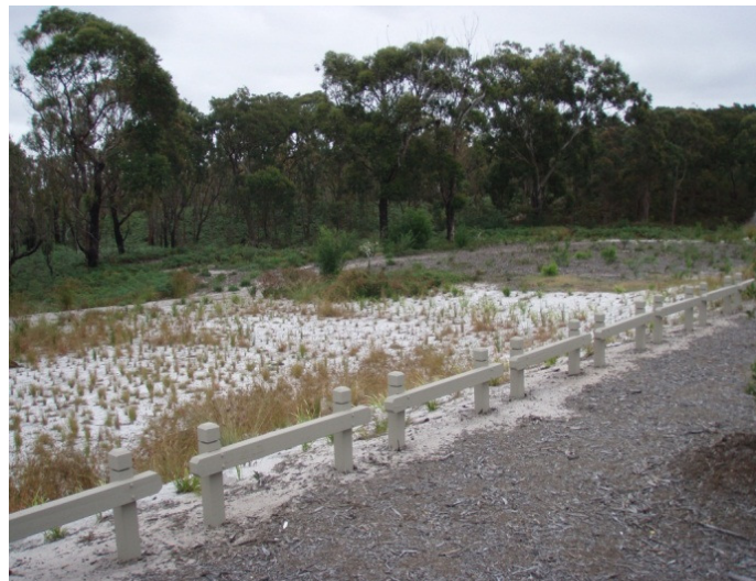
Figure 4-9 Typical Infiltration Basin
