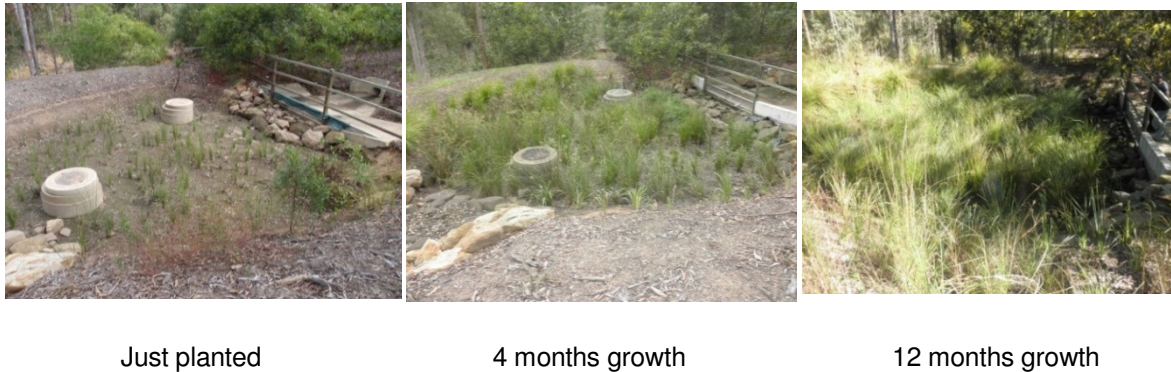
Figure 9-1 Example Bioretention Basin Establishment Photos
