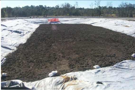
Biofilter media placed
