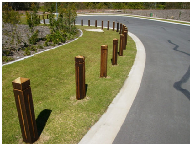
Figure 4-4 Typical Roadside Grassed Swale
