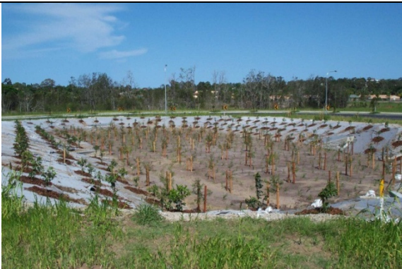
Biofilter planting completed
