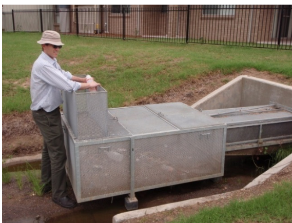
Figure 4-5 Typical Proprietary GPTs
