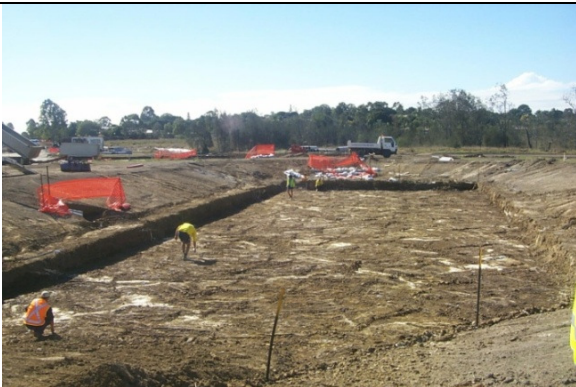
Excavation to biofilter base
