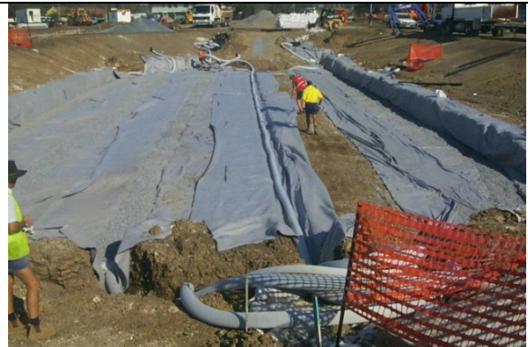
Placement of underdrains and impermeable liner
