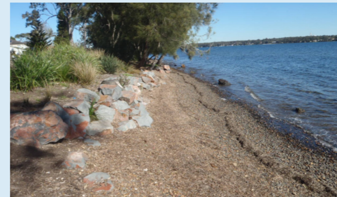
Revetment and native vegetation along lake foreshores. A combination of treatments – cobble beach, rock revetment and native vegetation – on a beach exposed to strong winds and waves. The combination of treatments allows a high level of protection from erosion, while retaining habitat and natural foreshore functions.
