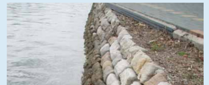
Seawall created without cement between the blocks to leave crevices, which provides valuable habitat (Source: Department of Environment and Climate Change NSW, 2009).
