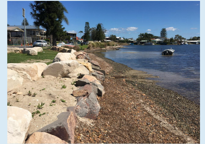
Combination of cobble beach, sand and rock revetment at Belmont.
