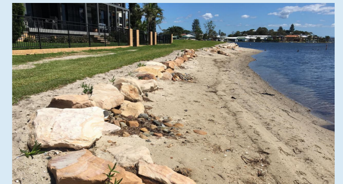
Combination of sandy beach and rock revetment at Belmont.
