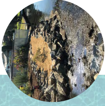
Saltmarsh & Rock Revetment © 2018 Lake Macquarie City Council
