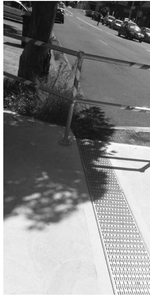
Example of a drainage grate on a kerb extension appropriate for a Neighbourhood Centre
