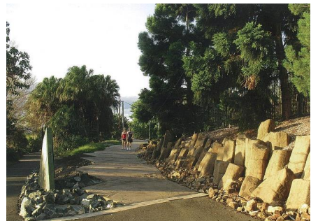
Large stacked boulders for informal retaining.
