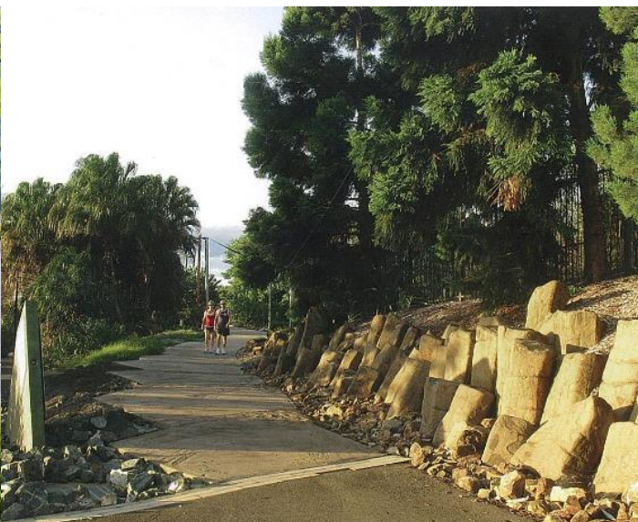
Image 2: Large stacked boulders as feature retaining to garden beds, maintaining the bush theme proposed for Mount Hutton.
