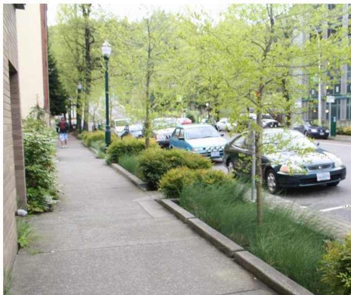
Image 1: Water sensitive urban design planter bed with street tree to verge.
