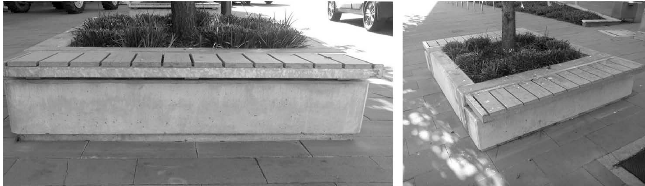
Existing precast raised planter on Pearson St, Charlestown
