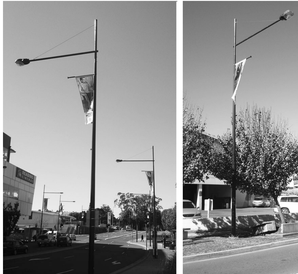
Existing street lighting with banner poles installed on Frederick St
