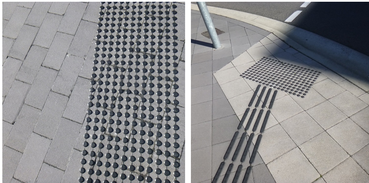
Existing bladed-shaft Hazard warning indicators on Pearson St Existing tactile indicators on the corner of Frederick + Ferris St.
