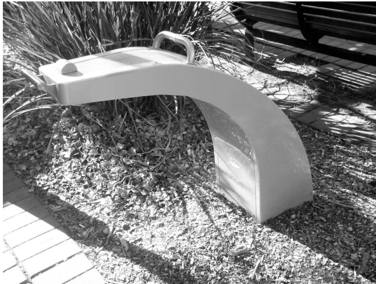
Existing cantilever style bubbler located in Charlestown Mall.
