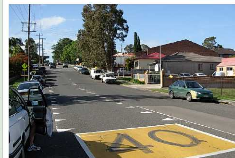
Smith St (south of Frederick St): 1200mm wide path to residential frontages both sides of the street.
