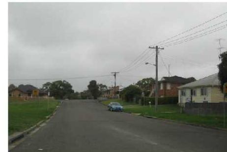
Dickinson St (eastern cycle by-pass around town centre)
