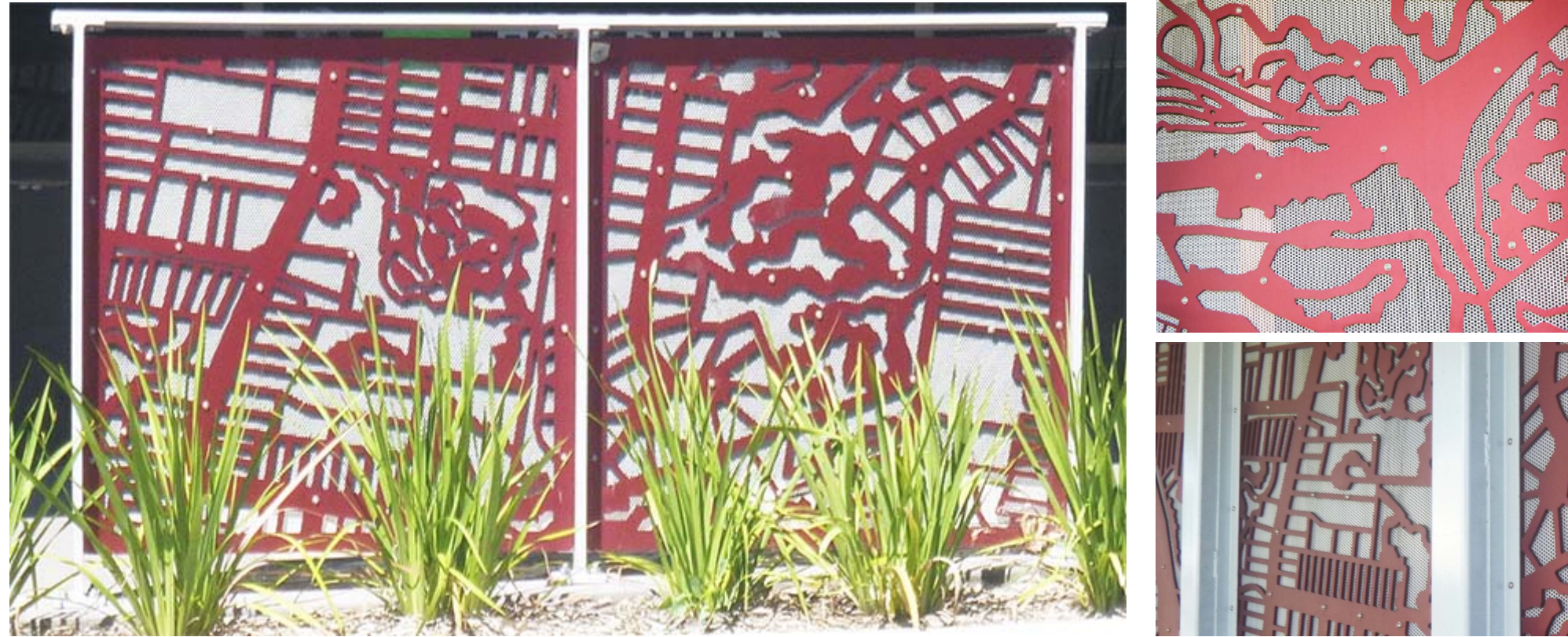
Example of Custom Balustrades installed at Main Rd Cardiff
