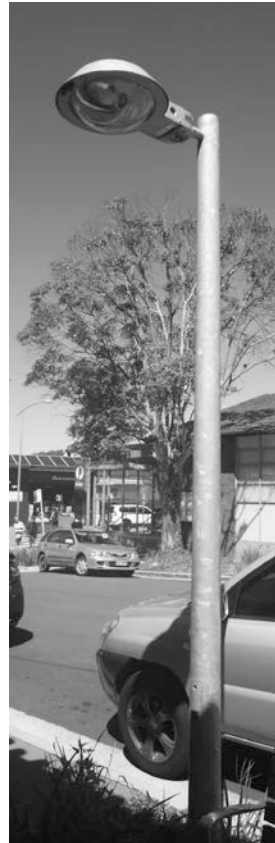
Existing pedestrian light pole, Veronica St
