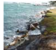
Pelican: active erosion occurring along the foreshore
