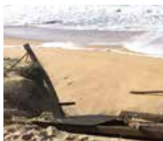
Damage to Blacksmiths Beach access as a result of storm surge, June 2016. Left unchecked other assets could be damaged or lost.
