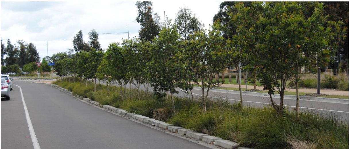
Figure 23 - Landscape planting in central median can provide a dual function for water management
