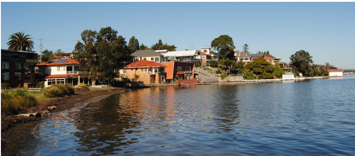
Figure 18 - Belmont Bay lake foreshore dominated by structures close to the lake edge
