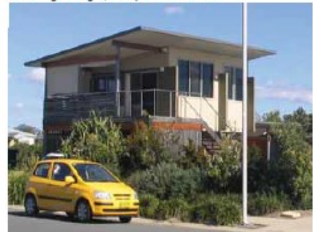
Landscape treatment to create privacy and hide underside of deck, also light weight material used within the building to breakup the buildform
