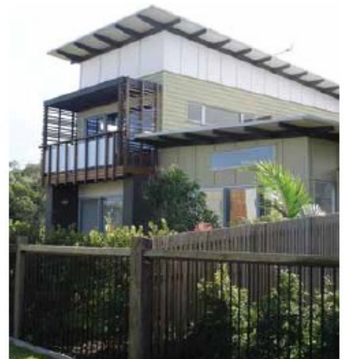
Articulated front elevation with light weight material to upper level and good eaves extension, sun shades / screens used to breakup facade
