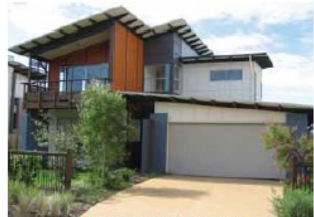
Articulated front elevation with clearly identified front entry balconies encouraged for views buildform and surveillance to the street
