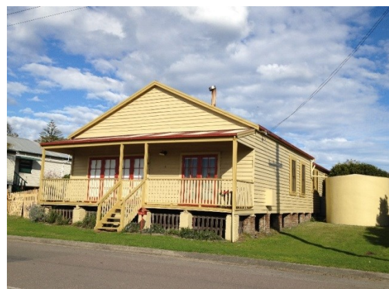
Figure 9 - Former Post Office and General Store
