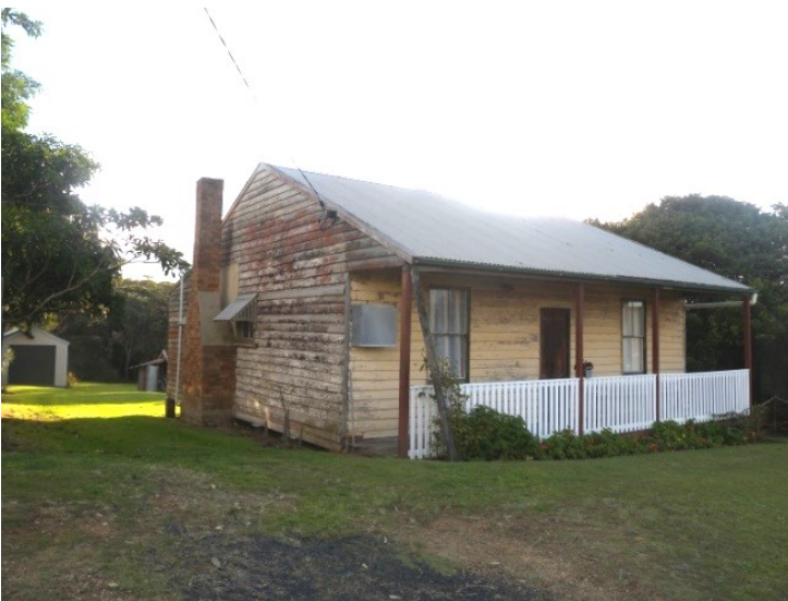
Figure 11 - Typical miners' cottage of Middle Camp
