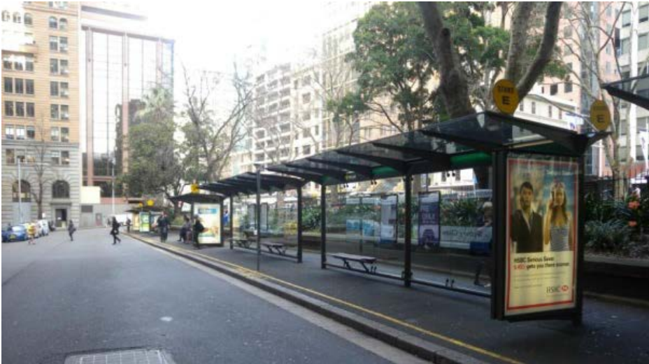
Figure 56 - High quality bus shelters with good shelter and visibility
