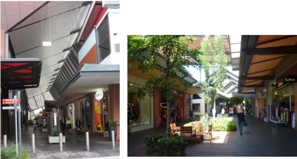
Figure 59 - Pedestrian lanes with natural air and light and specialty shops at footpath level.
