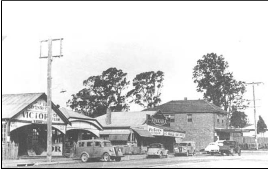
Figure 2 - Warners Bay Shopping Centre (Lake Macquarie City Library)
