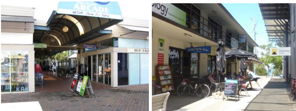
Figure 5 - Active links between car park and The Esplanade at Village Arcade and Bay Arcade (right)
