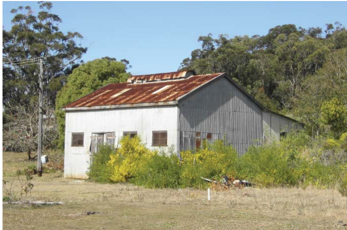
Figure A1.6.1- Existing former workshop building
