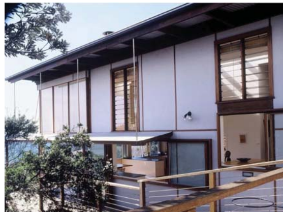
Figure A1.6.6 - Lightweight construction with timber detailing.
