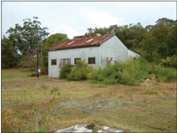
Figure A2.6.2 - Former workshop
