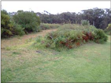
Figure A2.6.4 - Railway embankment
