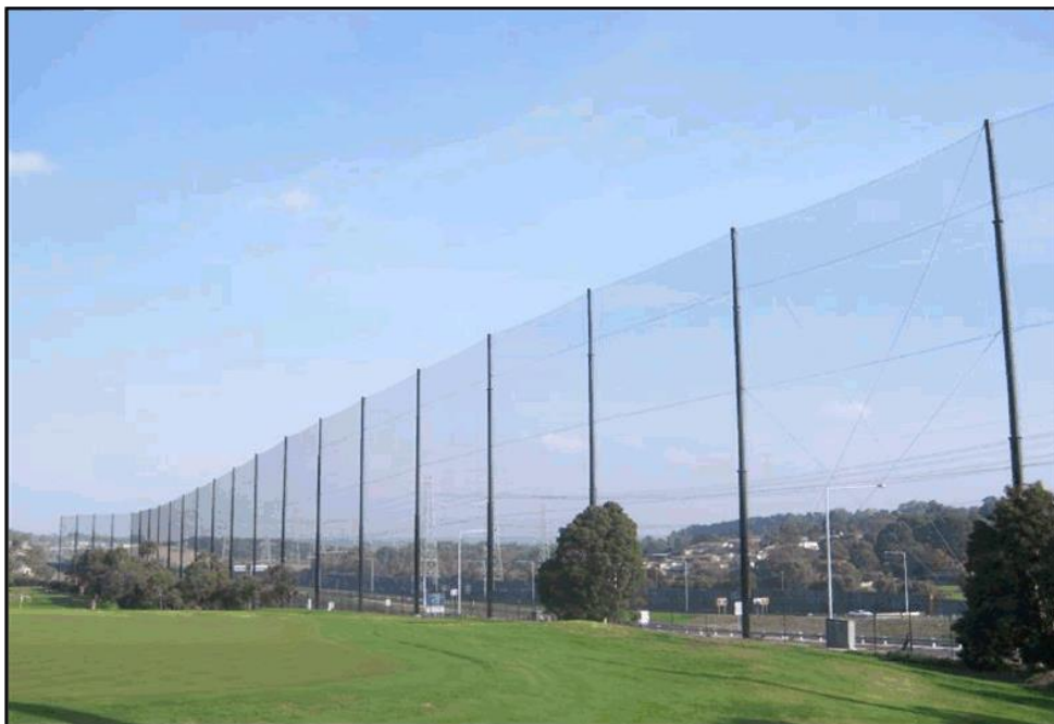
Figure 2 Example of 30 metre safety fencing at Ringwood Golf Club (source: CCI Safety Fencing)
