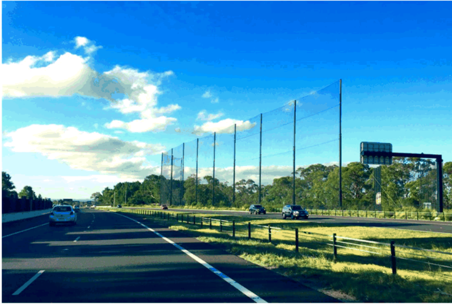
Peninsula Link – Melbourne – Comprising 2 screens on Centenary Park Golf Course at 30m tall and 400m total length adjacent to Peninsula Link Freeway.
