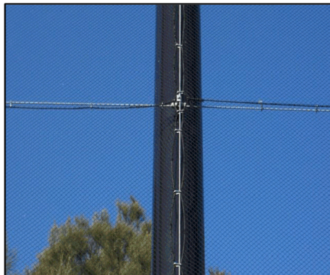
Figure 5 Example of wire rigging fittings (source: CCI Safety Fencing)
