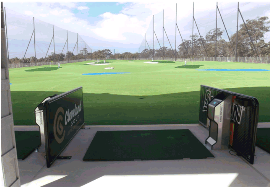
Thornleigh Golf Centre - Sydney. Despite the engineering complexity created by not allowing pier footings into the ground due to it being a clay capped site over an old tip, it was stipulated by Council that a screen of not less than 36m be erected to protect from errant balls going onto the the adjacent Pennant Hills Road to the south (right side of the range).
