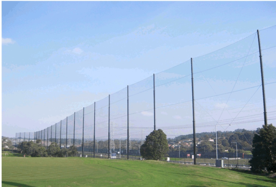
Ringwood Golf Club/Eastlink - At 30m tall this is one of the highest and certainly the longest engineered high safety screens in Australasia
